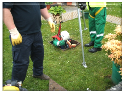
Culvert inspection with Draintech Services Ltd
